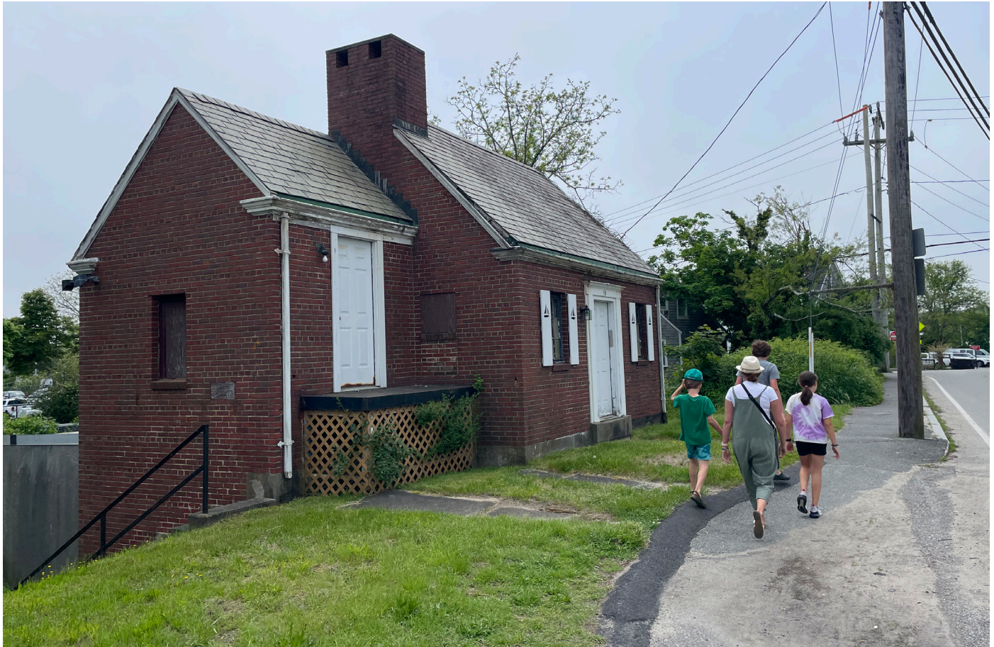
Figure 10: Building at 91 South Street
