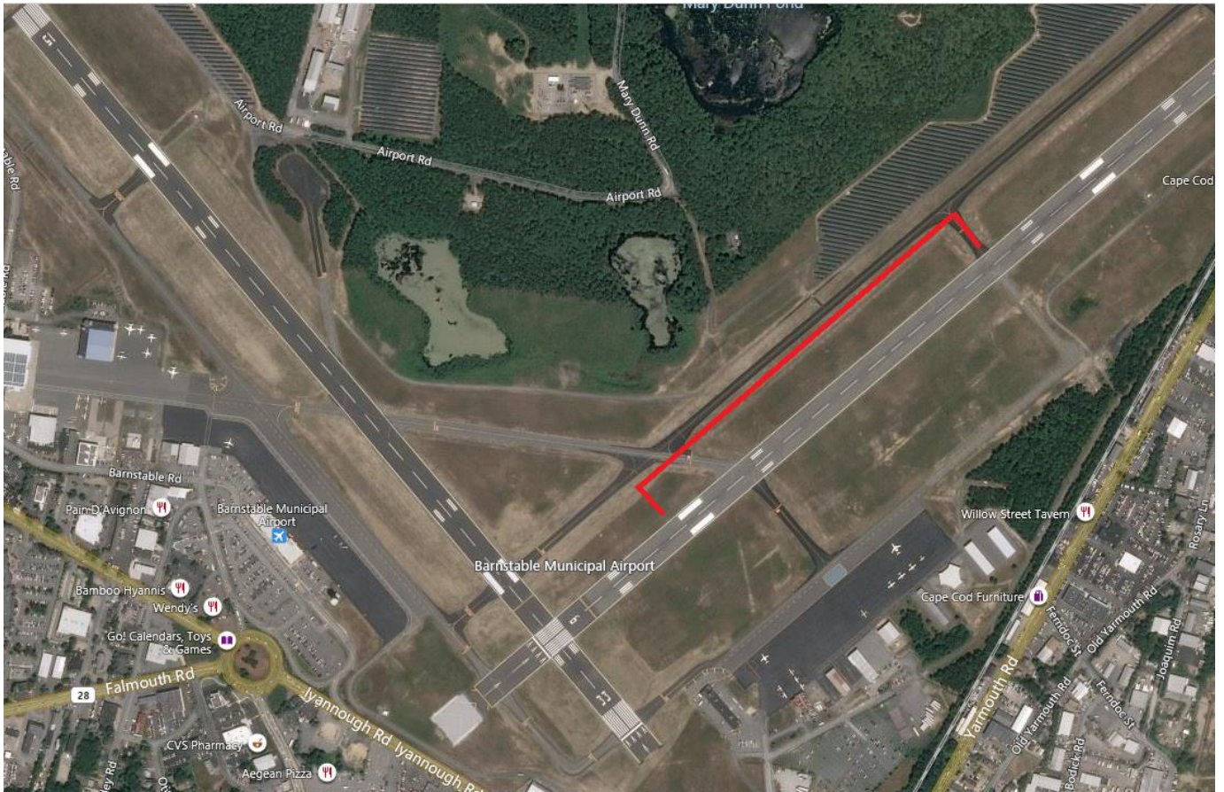
Portion of Taxiway Bravo
