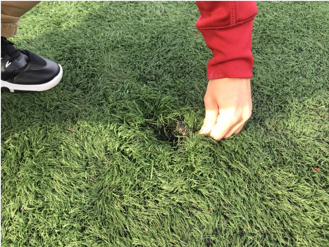
Barnstable High School Synthetic Turf Replacement
