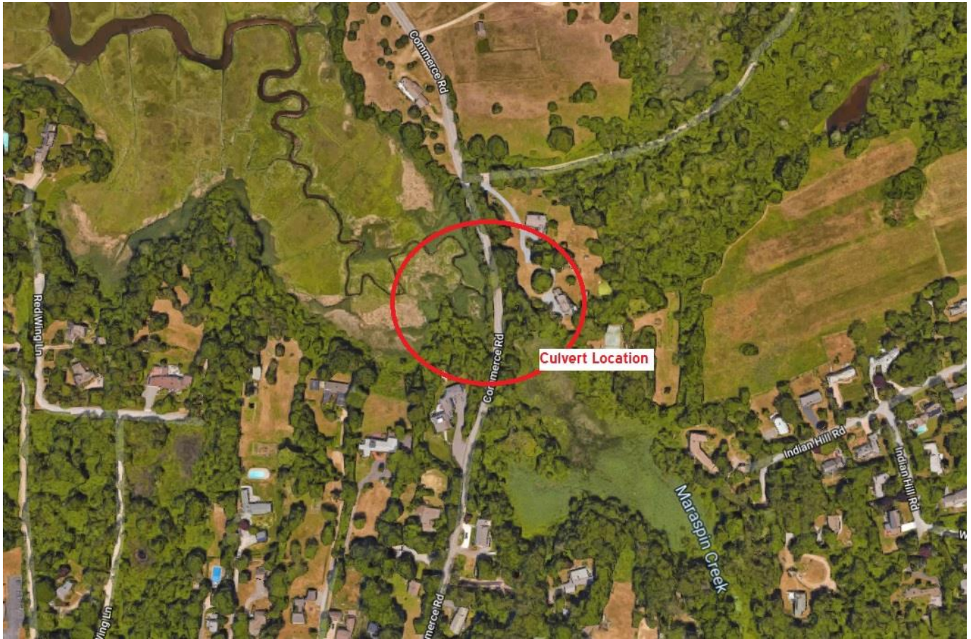
Commerce Road Culvert
