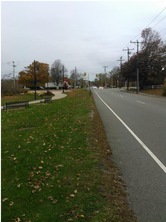
Sidewalk Installation: Bumps River Rd Centerville, Main St Cotuit, South St Hyannis
