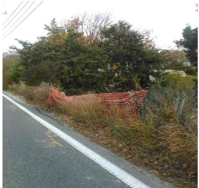
Snows Creek Culvert
