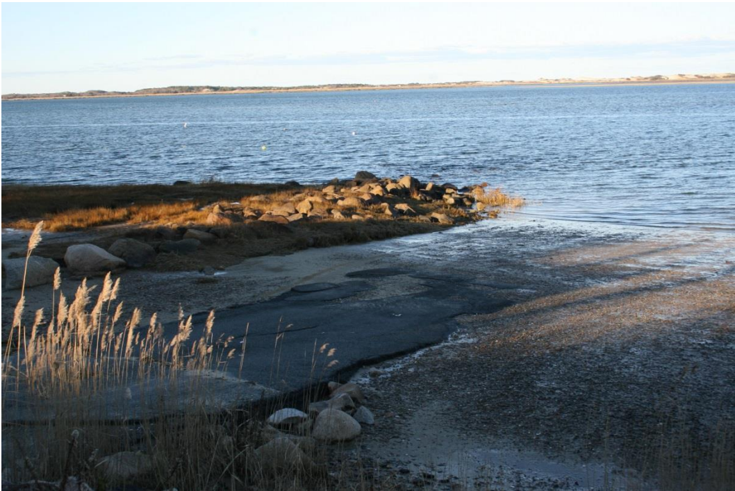
Scudder's Lane Boat Ramp
