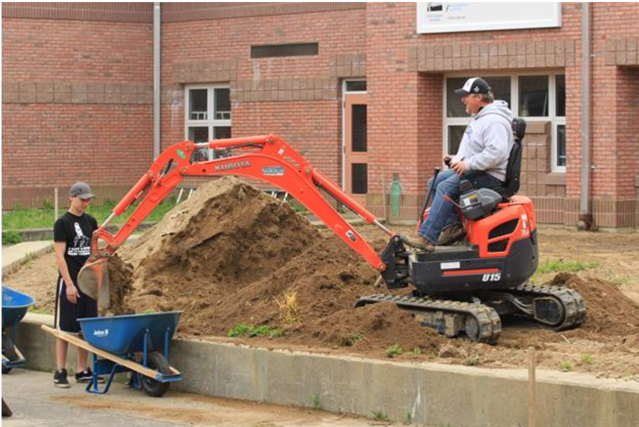
Barnstable Unit Elementary Courtyard Improvements
