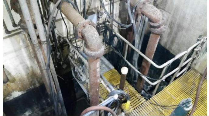
Old Colony Pump Station Wet Well
