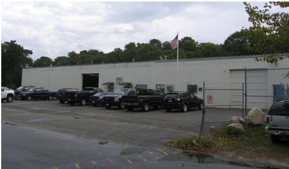
Facilities Maintenance Shop
