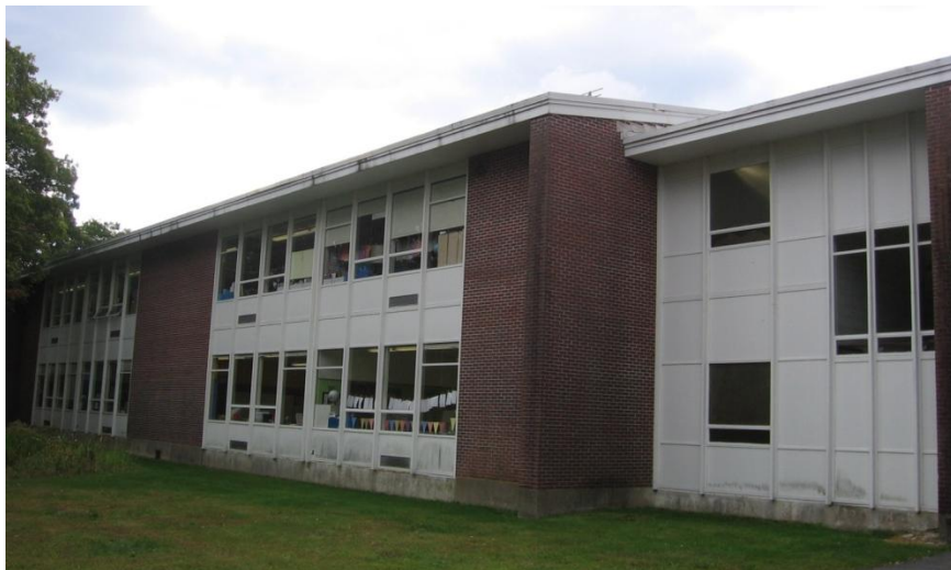
Windows needing replacement
