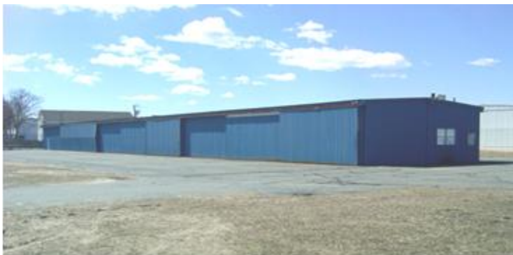
Existing T hangar
