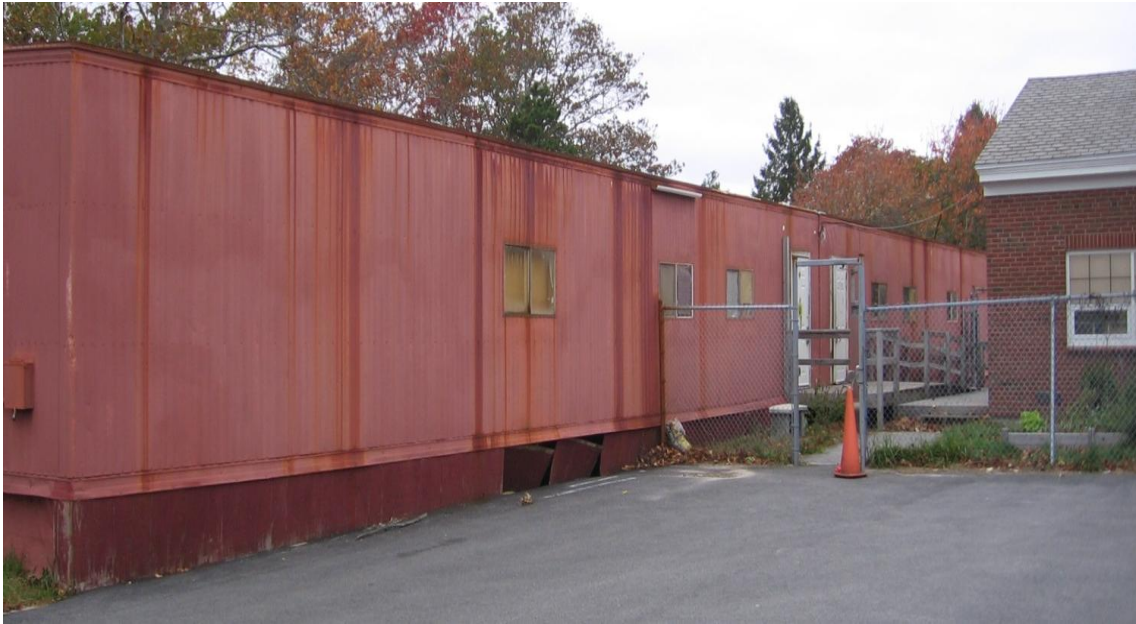
Typical Portable School Building
