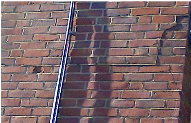
BCHMCPS Roof & Façade Replacement (Cracked Mortar, Bulging Wall)
