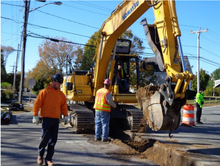
Replacing Water Pipe
