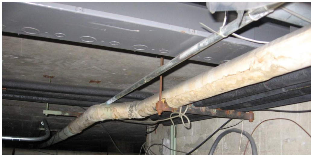
Typical Asbestos Covering Pipes
