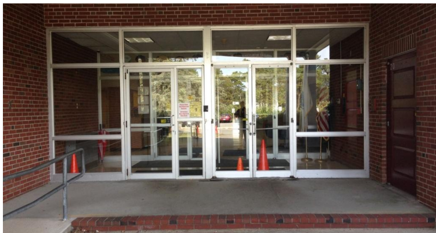
HYW Interior/Exterior Door Improvements
