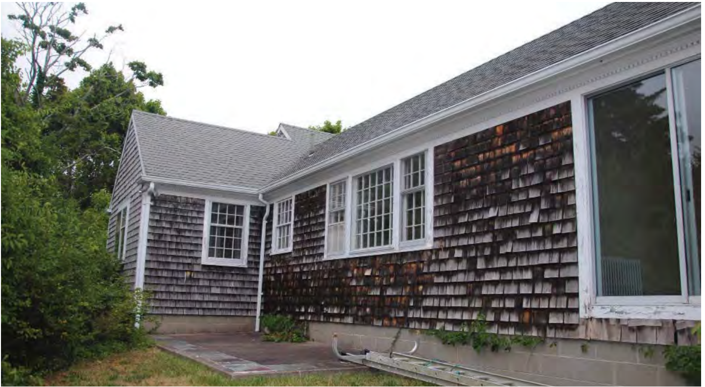
VIEW OF EAST ELEVATION (RIGHT FROM FRONT)
