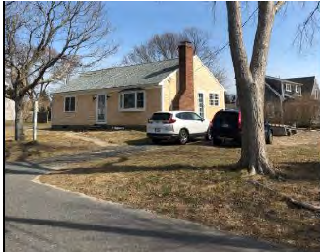
Right View from Street. Panels not visible.
