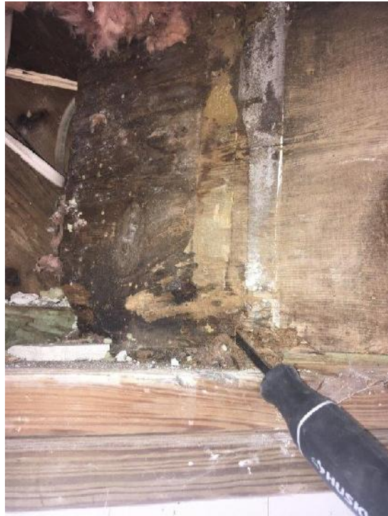
Typical second floor wall top plate & third floor beam with rot/deterioration at exterior wall support top plate; no mechanical fasteners observed or no longer engaging framing
