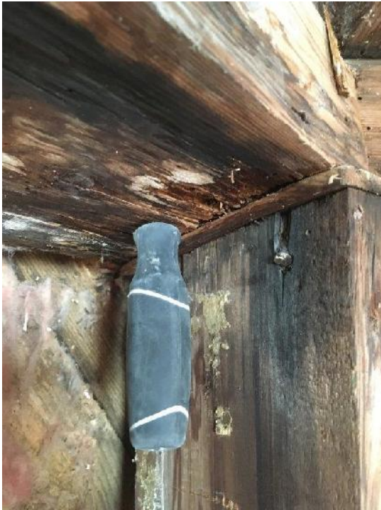
Typical second floor wall top plate & third floor beam with rot/deterioration at exterior wall support top plate; no mechanical fasteners observed or no longer engaging framing
