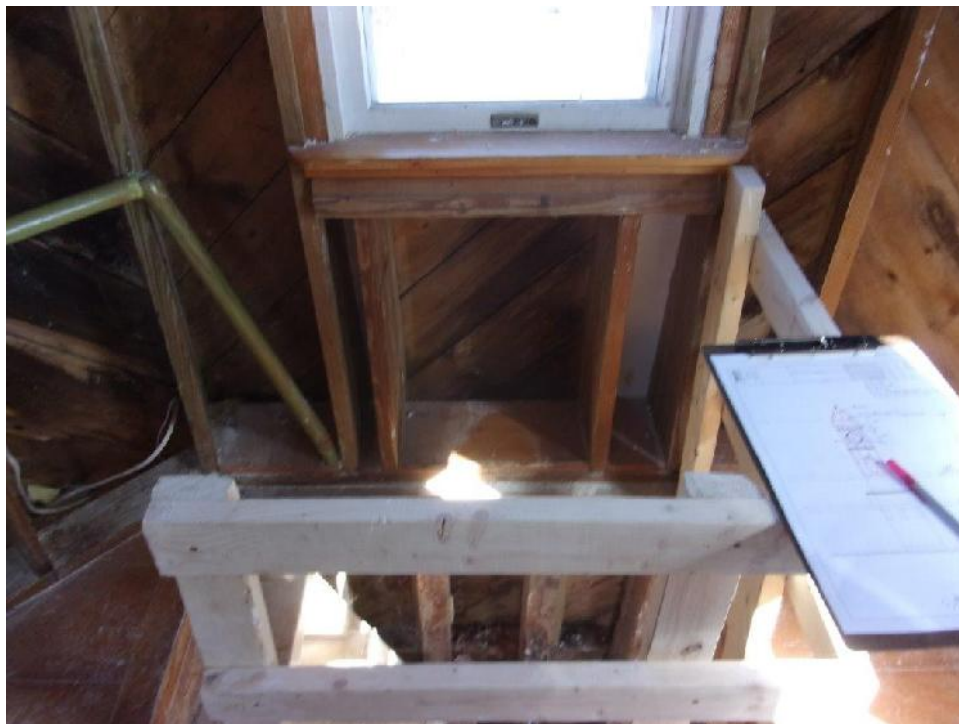
Typical third floor window sill framing
